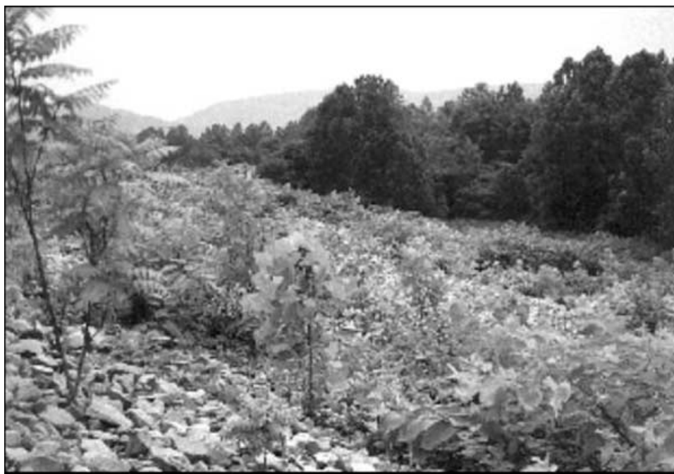
Fig. 4. Sycamore, tree-of-heaven, and Japanese knotweed growing on a disposal cell cover. Root intrusion increased the hydraulic conductivity of the compacted clay layer by two orders of magnitude.
